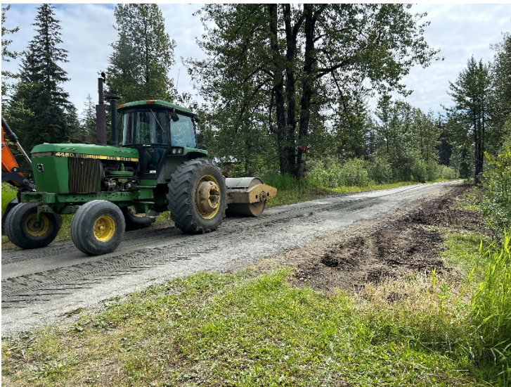
Glen's Ditch Road Improvement
