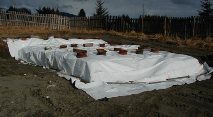
Balefill with poly tarp Alternate Daily Cover (ADT) Representing Winter 2008-9 use Measures 20' x 60'
