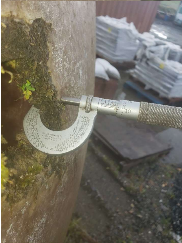
Outer tank wall thickness measurement.
