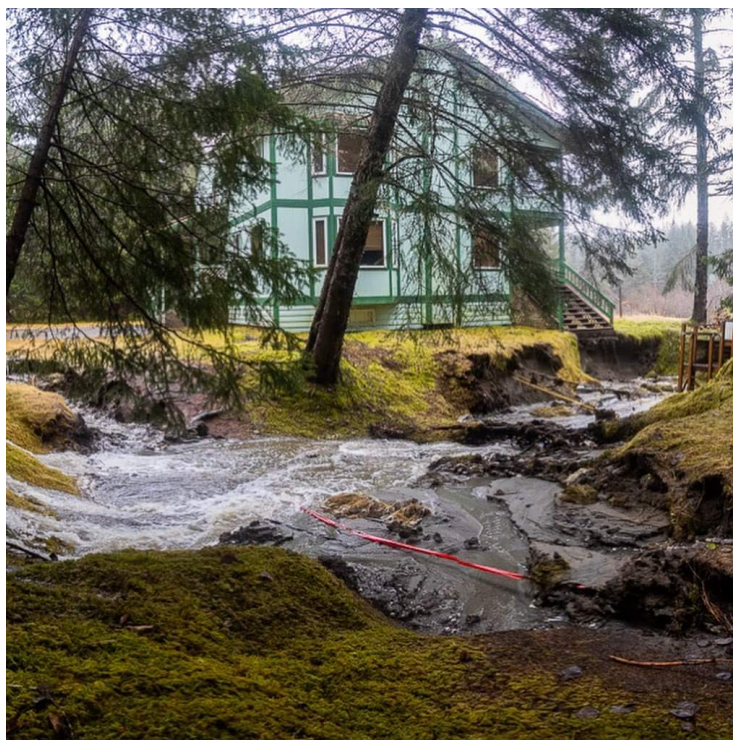
Figure 13 - Erosion near home on River Bend Drive
