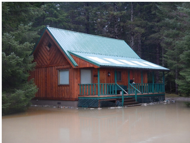
Figure 10 - Flooded Home on Wilson Road (December 2020)
