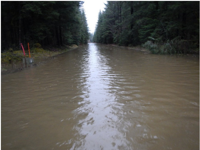
Figure 1 - Wilson Road Flooding near Hemlock Road (December 2020)
