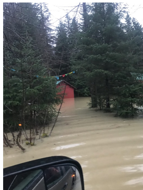
Figure 11 - Chase Driveway Flooding (December 2020)
