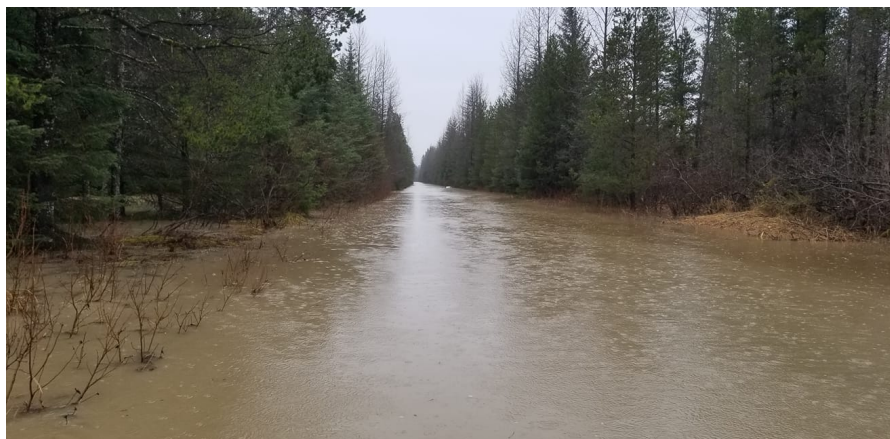
Figure 3 - Wilson Road Flooding Near Chase Drive (December 2020)
