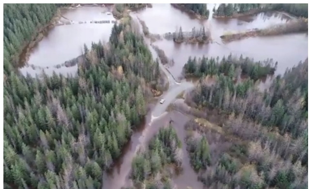
Figure 5 - Wilson Road Flooding Near Gravel Pits (October 2018)
